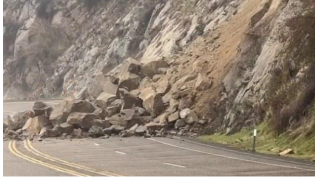
54 - 2023 Rockslide HWY 168 Fresno County
