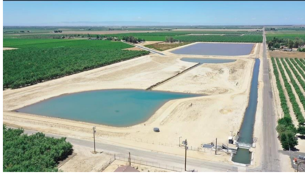
25 - Central Basin site at W. Central Ave and S. Hughes Ave was completed in 2021, with operations beginning in 2022 - Fresno Irrigation District
